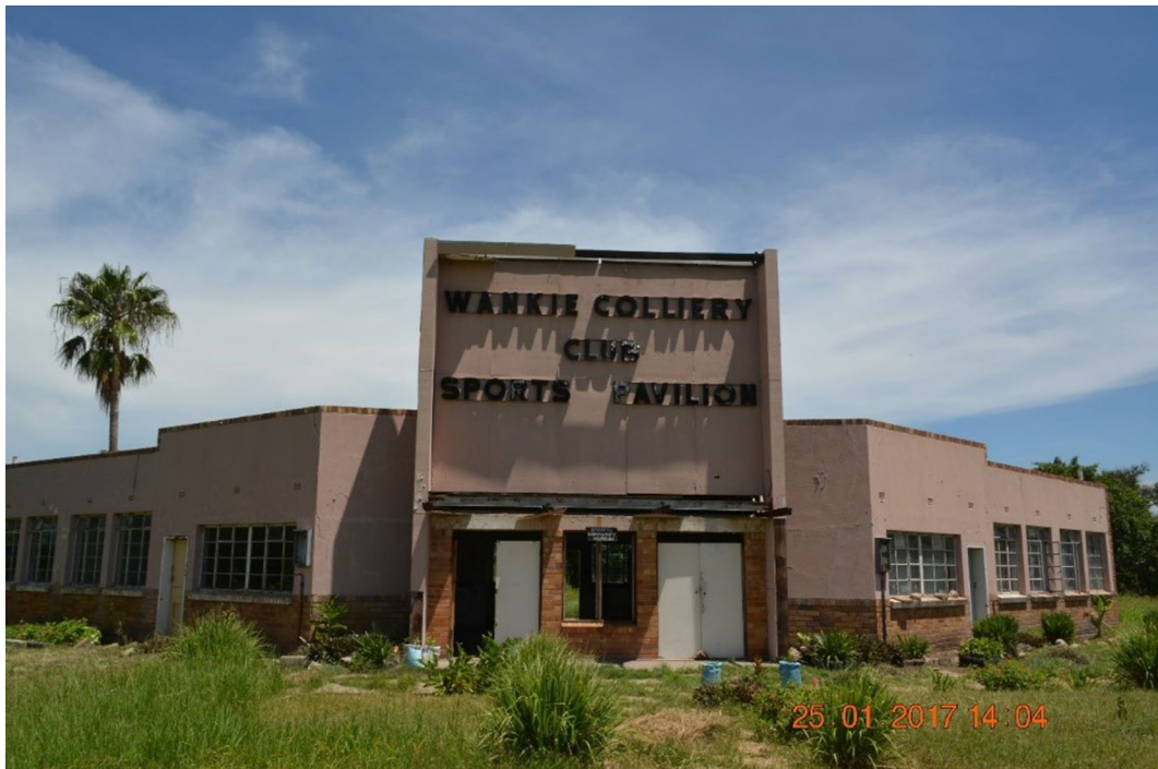
Figure 2. The donated pavilion building prior to renovation. Photo courtesy of the author (Munyaradzi Elton Sagiya).
