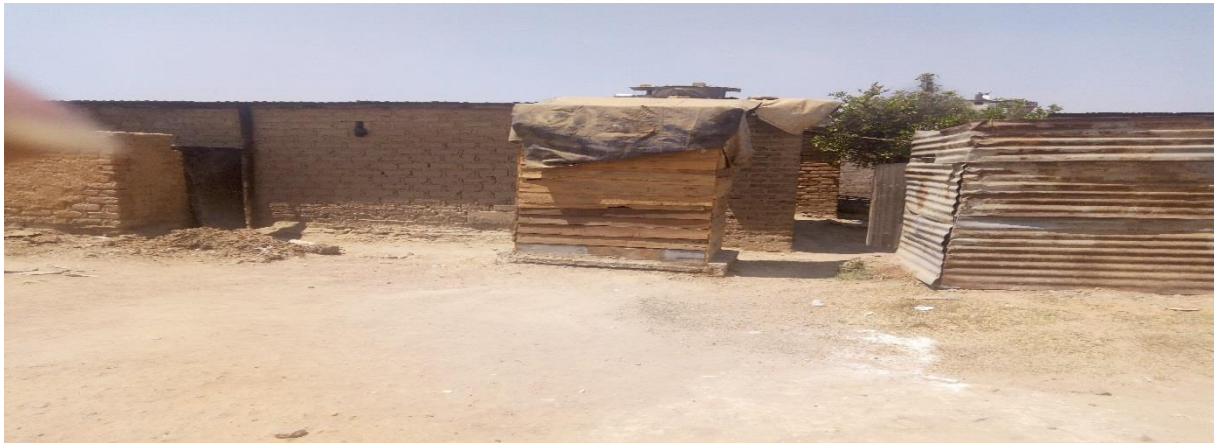
Figure 4.5 Shelters in Epworth.
